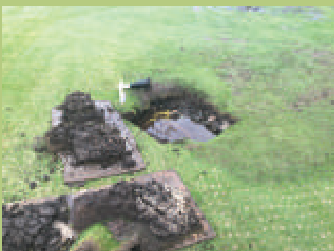
Another leak on #1 fairway
