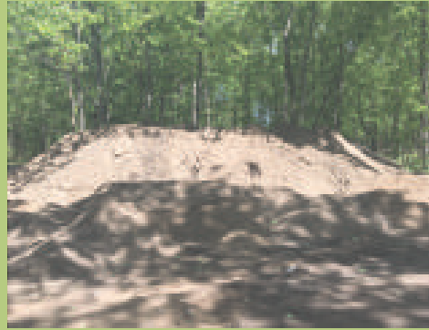
Material removed from XGD Drainage Project
